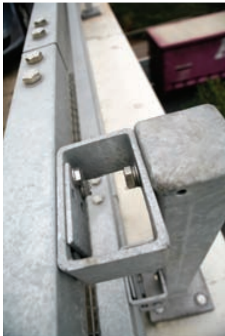
Detail of Normal Containment Parapet support section
