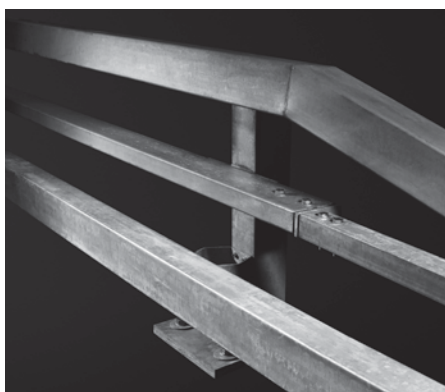
H4a unclad parapet transition
