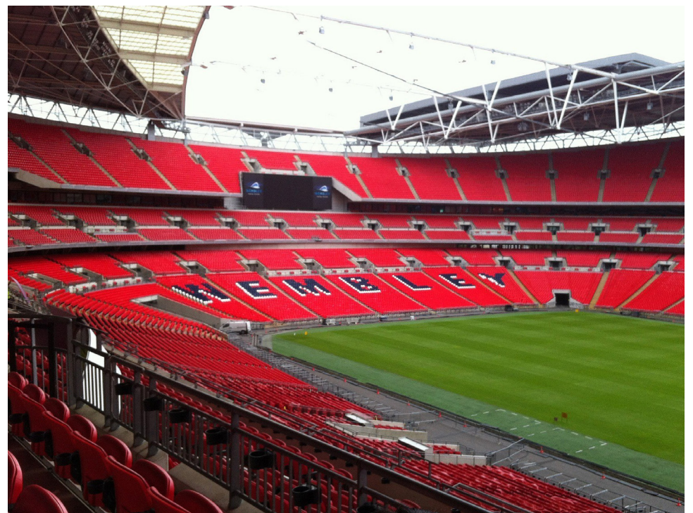
The iconic Wembley Stadium contains 22,000 tonnes of steel from Hartlepool and Corby – but it's not just the UK's capital where our steel can be found. It can be seen in recognisable structures worldwide.
