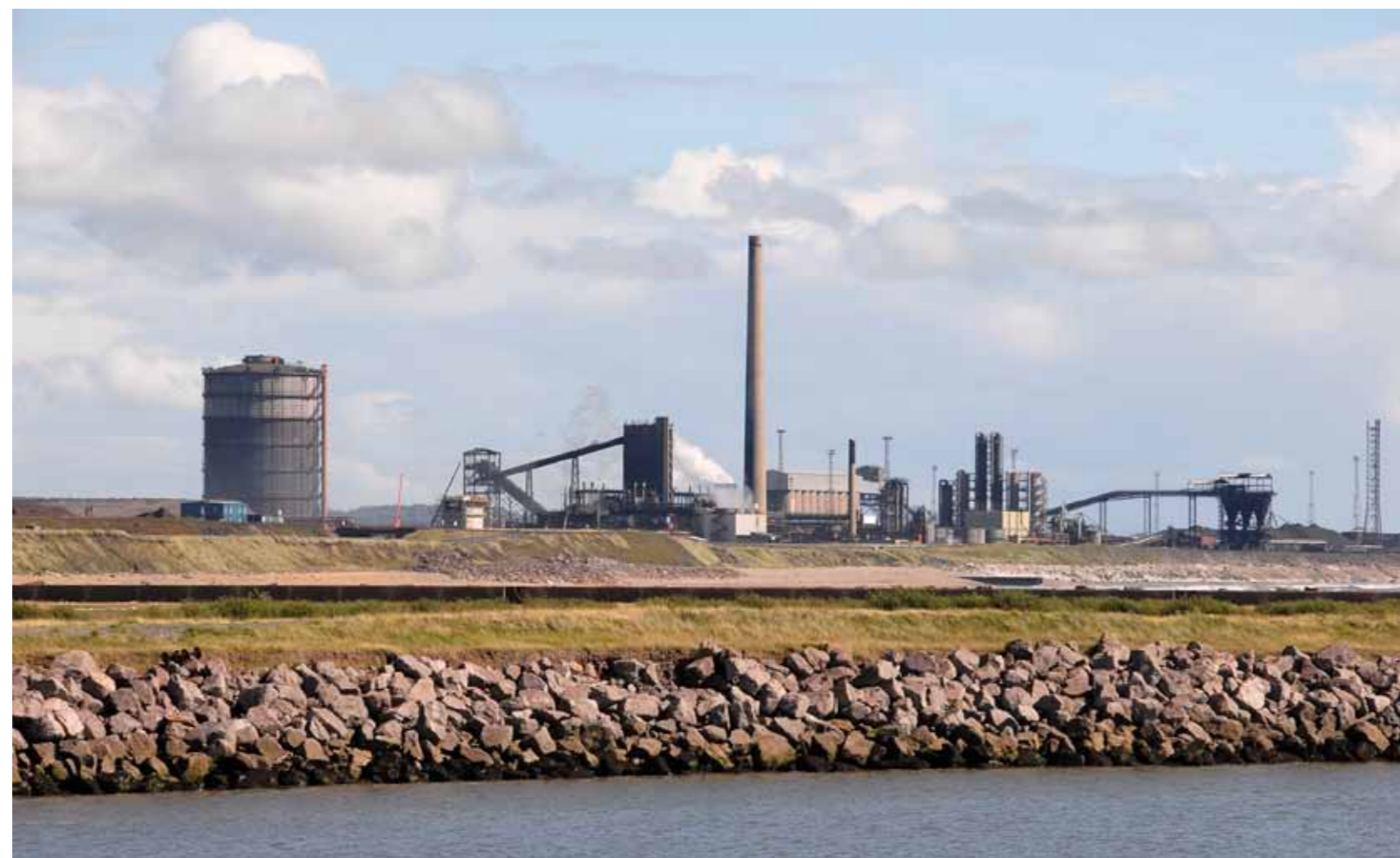
A new extraction hood at Morfa Coke Ovens will improve the plant's environmental performance
