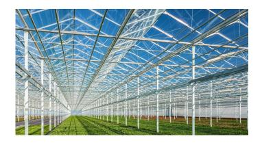
Ensuring quality in every piece, the reliable performance of our cold formed welded steel greenhouse horticulture tubes allows you to process with confidence in automated robot production. They are usually supplied in accordance with EN10219, in either S235JRH or S275J0H. However, we can also provide other steel grades such as S355J2H or S500MH. The utilisation of higher strength steel grades can, for example, have a beneficial effect on the durability and longevity of rail systems.
